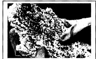
[Mold growing on a piece of ceiling tile]
